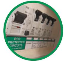
**2** Fusebox incorporating an RCD. This is the safest form of RCD protection and should be tested quarterly.
